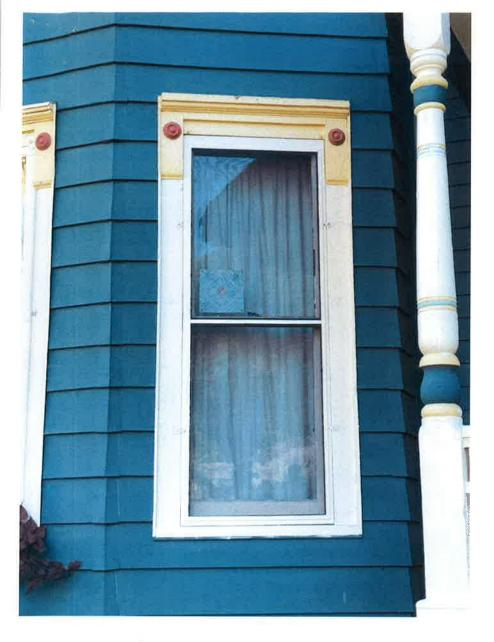
This is an original window. The vinyl window in the parlor will be replaced with a window that matches this window in size and design. It will be longer and wider than the vinyl window, double hung and wood interior and exterior. The replacement window will also have exterior trim updated to match this window.
