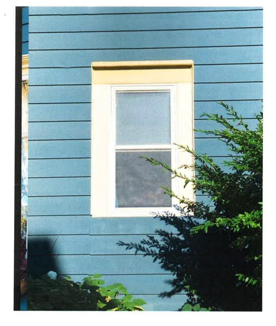
Existing exterior window is currently vinyl and shorter than original. We plan to replace this window with a longer, wood double hung window that matches the original windows. See the following photos for original windows.
