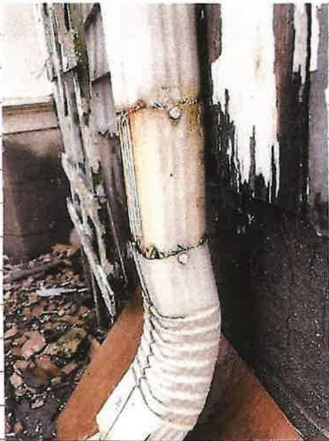
The gutter system is approximately 30 years old and in bad shape. On this one, the water is running down behind it along the siding. I put a piece of plywood at the bottom to divert it a little bit away from my limestone foundation. I would like to replace it with the same materials.
