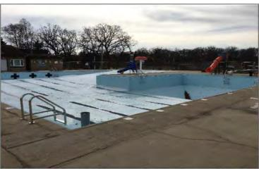
The top of the pool wall and gutter exhibit some deterioration. This should be monitored for future repairs (see photos below). The interior finish of the pool is paint. A new coat was installed this past spring after several repairs of concrete cracks and expansion joints. Repairs of this type will be required more frequently as the pool ages.
