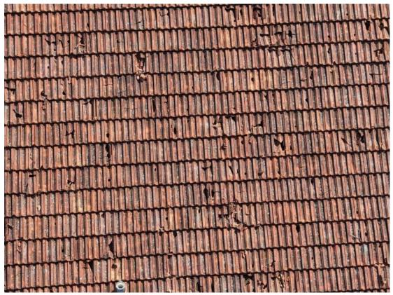
Figure 2 - Close-up of hail damage
