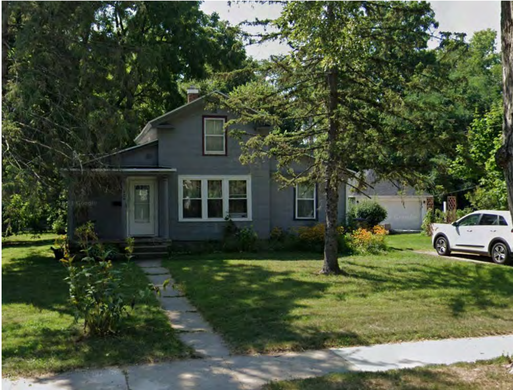
325 W Main Asbestos Cement Board Siding
