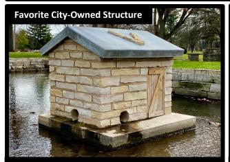
**Leonard-Leota Park Duck House** Spring floods and high water in the West Lagoon compromised the foundation of the Duck House, the unique and beloved structure was rebuilt on a robust foundation with original roof details and replica door.
