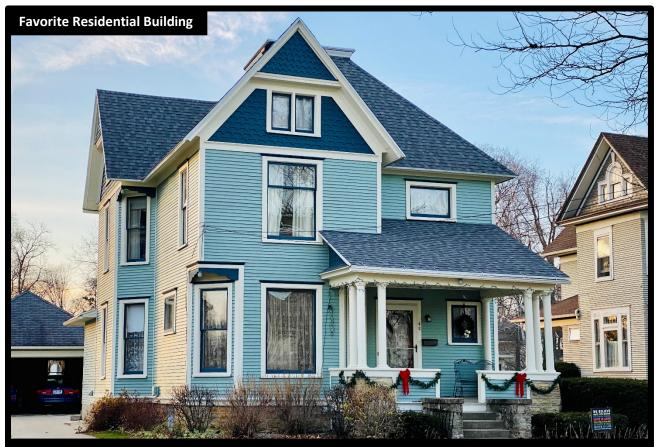
**45 N First Street** Exterior renovations included removing aluminum siding to uncover and restore the original wood siding and restoring the original open front porch.
